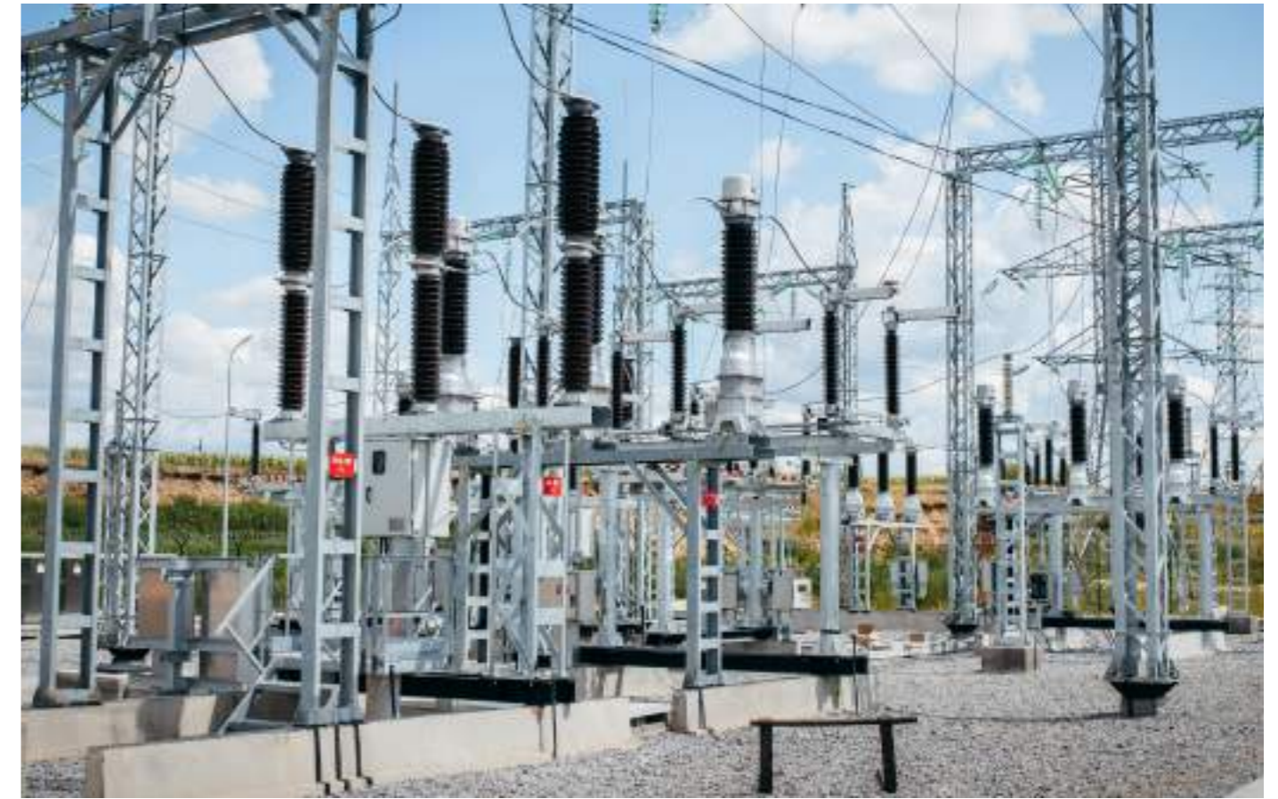
Figure 8: Hydrogen generation equipment at substation
