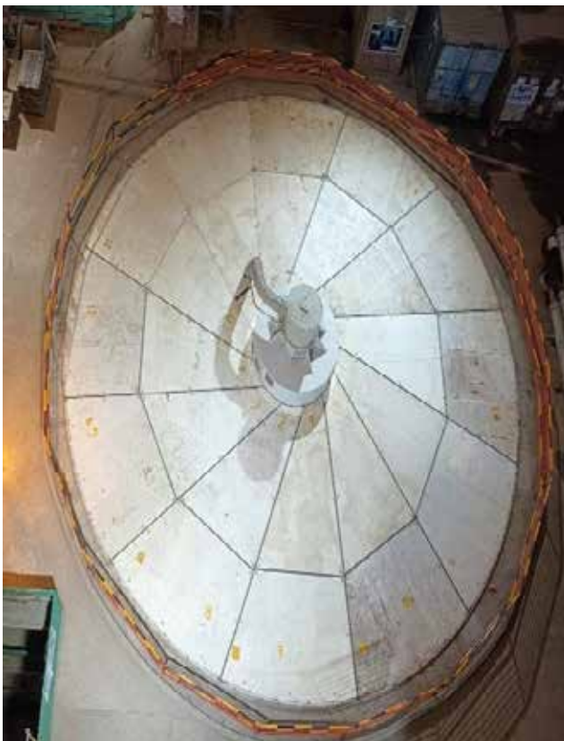
BOXING UP OF UNIT#1 & UNIT#2 (250 MW EACH) COMPLETED – 2000 MW SUBANSIRI LOWER (ARUNACHAL PRADESH)
