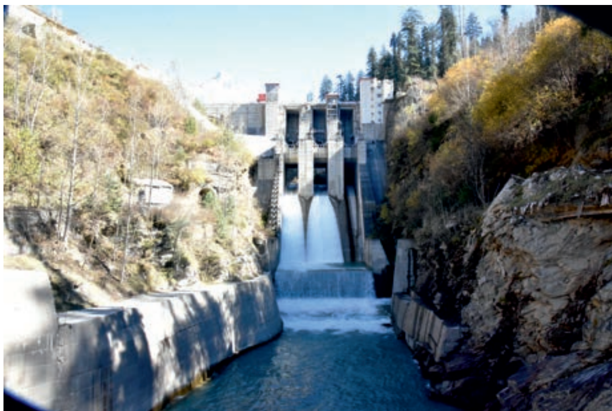
800 MW Parbati-II Project (Himachal Pradesh) – Dam
