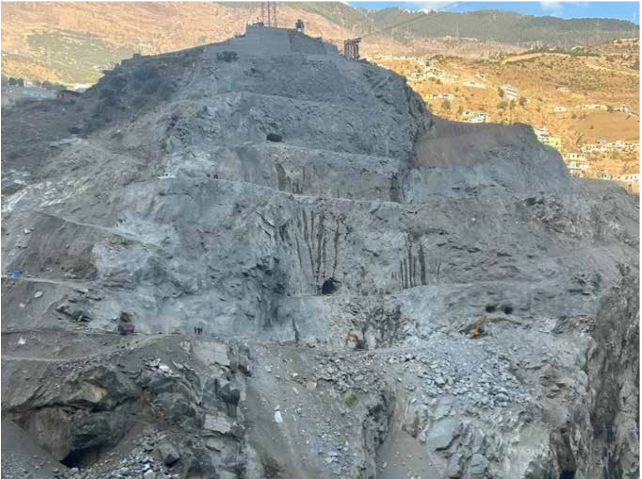
DAM ABUTMENT STRIPPING- 850 MW RATLE (UT OF J&K)
