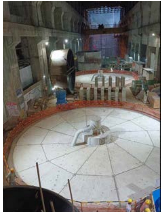
BOXING UP OF UNIT#1 & UNIT#2 (250 MW EACH) COMPLETED – 2000 MW SUBANSIRI LOWER (ARUNACHAL PRADESH)
