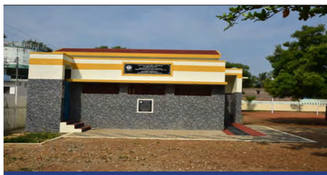
Construction of toilet blocks near Kudankulam at Tamil Nadu
