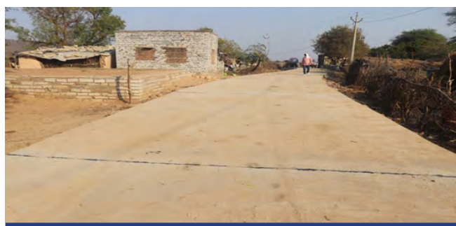
Construction of concrete road, drainage, footpath, culverts etc. near Rawatbhata at Rajasthan
