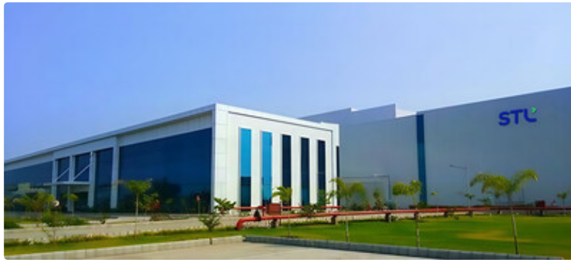
STL's Industry 4.0-enabled Glass Preform manufacturing facility, Chhatrapati Sambhaji Nagar, Maharashtra.
