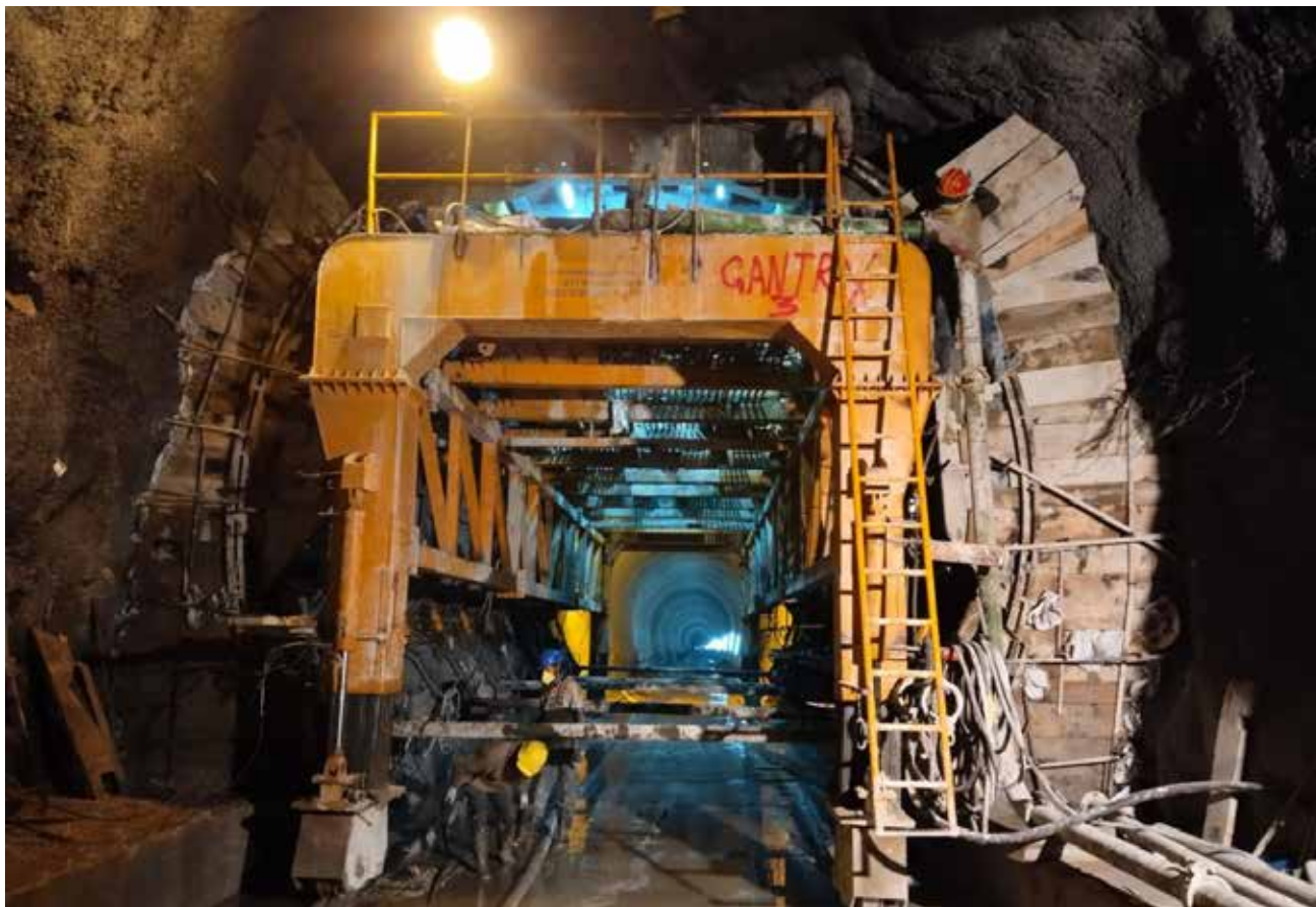
LINING WORKS IN FACE-3 & FACE-4 OF HEAD RACE TUNNEL – 800 MW PARBATI-II (HIMACHAL PRADESH)
