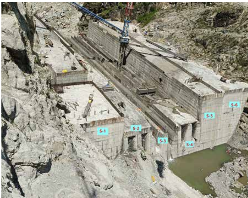
CONCRETING OF 135 M HIGH CONCRETE GRAVITY DAM – 624 MW KIRU (UT OF J&K)
